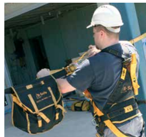
Web temporary life line, ratchet tensioning method.
